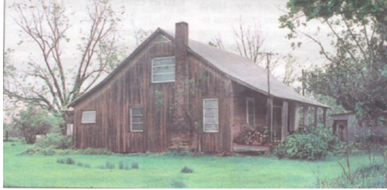
The home Claude Davis now lives in was built in 1868. It is a sturdy monument to the skill of the builders. The current owner maintains it and a hand-hewn barn.
